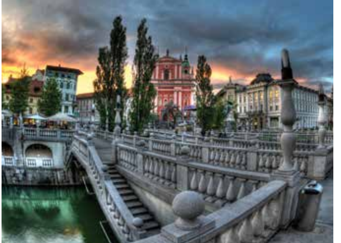
Triple Bridge / Tromostovje
